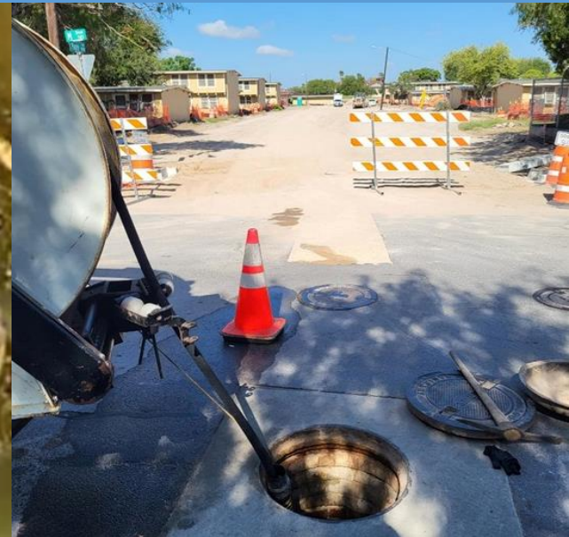
Clearing a Sewer Backup
