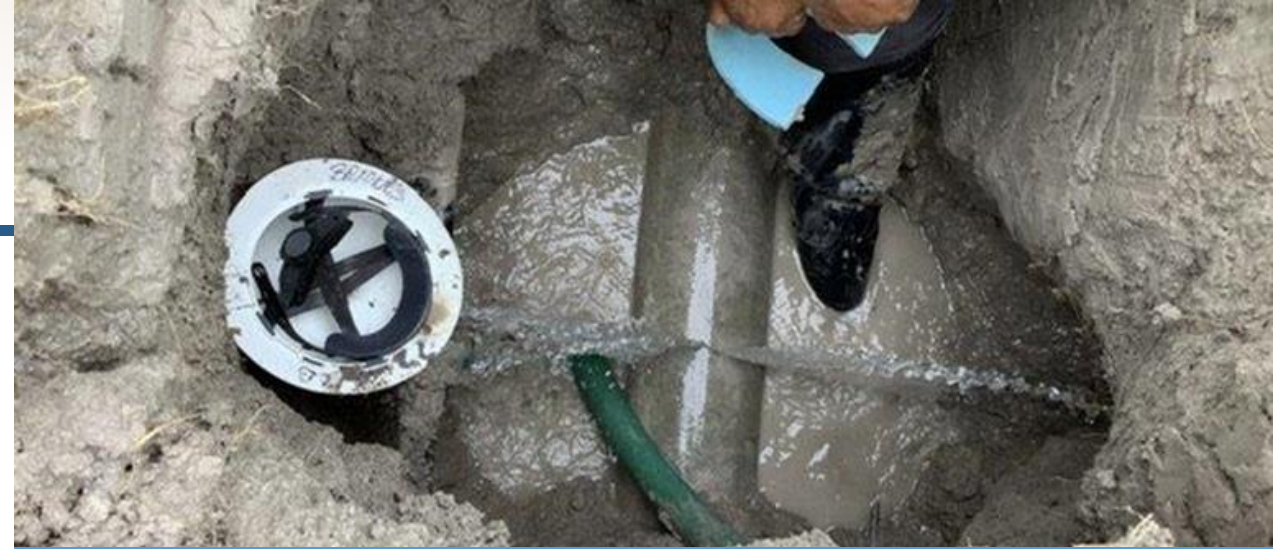
Repairing an Active Leak
